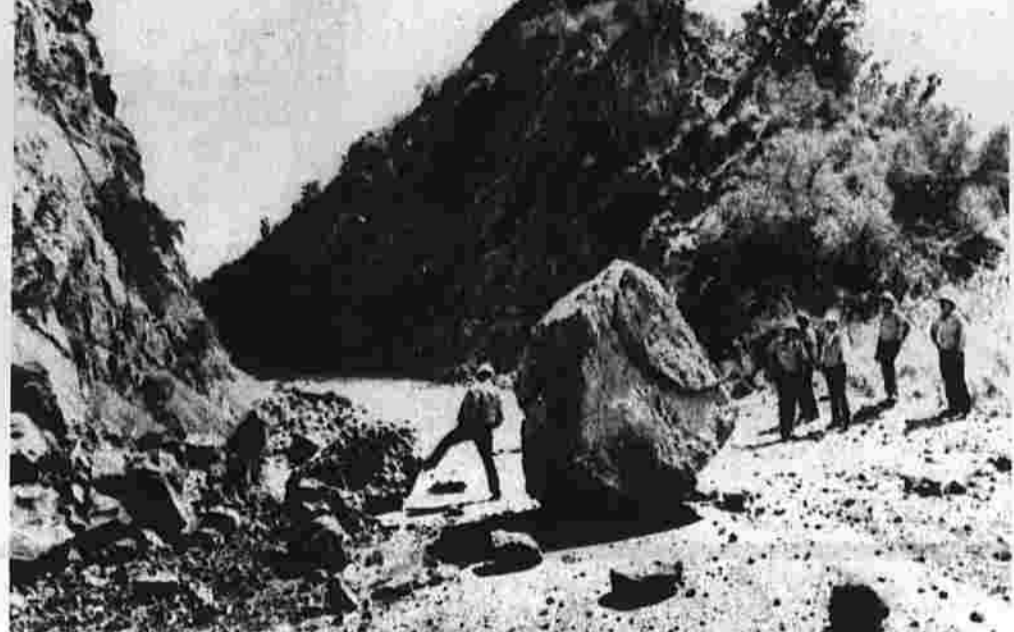
California road crew surveys rubble blasted from hillside in the San Marcos Pass north of Santa Barbara Monday. The outcropping, loosened by Sunday's earthquake, threatened to drop onto the highway and had to be removed. (UPI photo)
